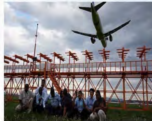
CNS system Maintenance Course : July 2014
